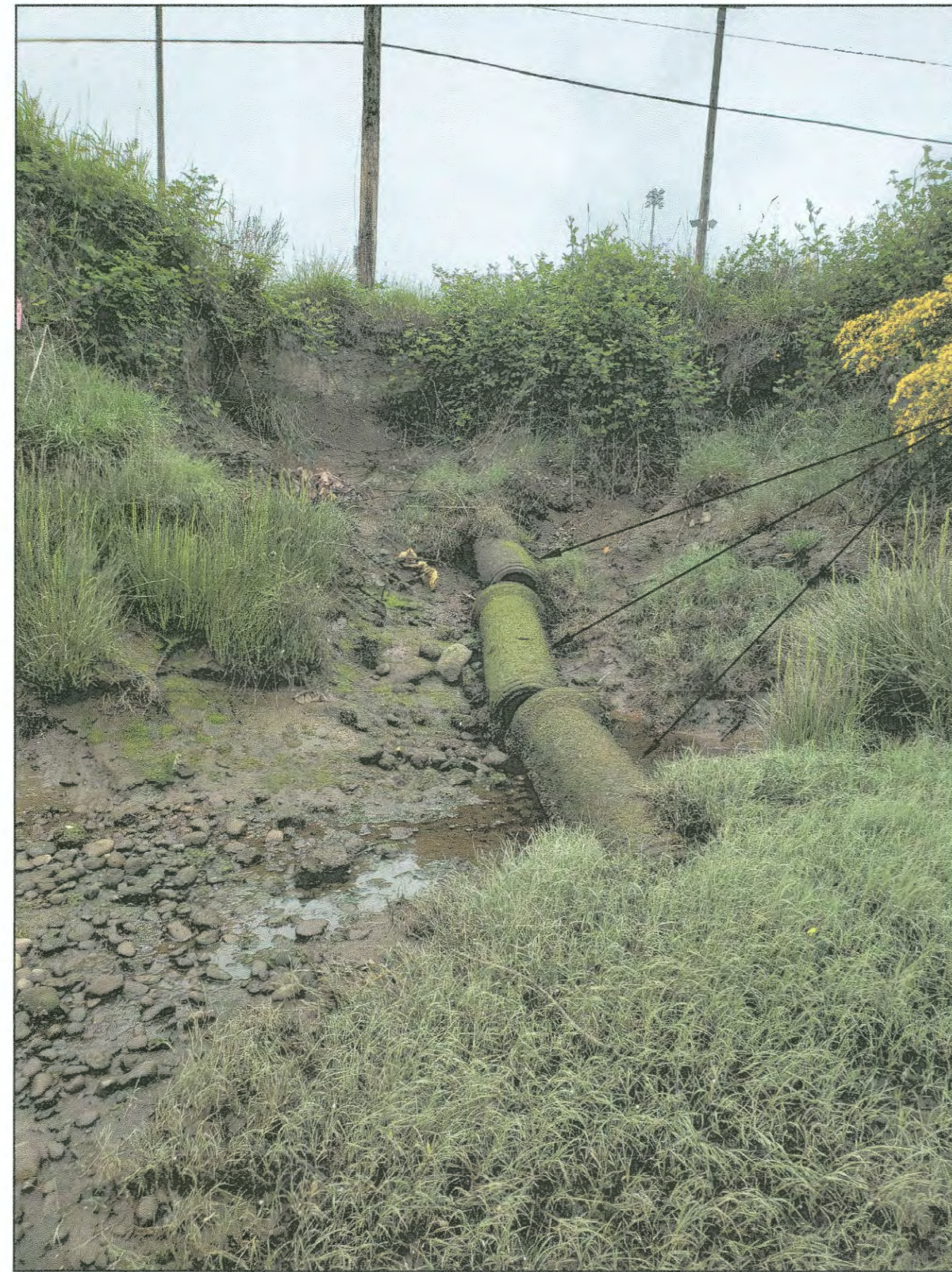
3 OUTFALL EXISTING CONDITION PHOTO
